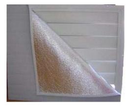
3. Peel the opposite side of the release liner off. Attach the piece of insulation (silver side towards shutter) onto the Velcro, leaving an overhang on all four sides. Firmly rub the insulation in to the Velcro to get a good bond.
